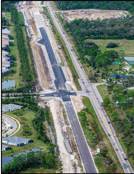
Southbound Paving at Observation Boulevard
